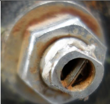
COMPONENTS AND LEAKS
